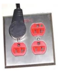
Red outlets indicate emergency back up power. Will automatically go to generator in the event of a power failure. Electrical equipment must be checked annually by BIOMED- always confirm sticker is in date
